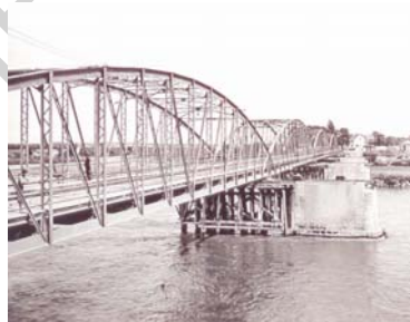
Figure 1. Sava bridge in Zagreb (1938.), a bridge constructed solely by welding
